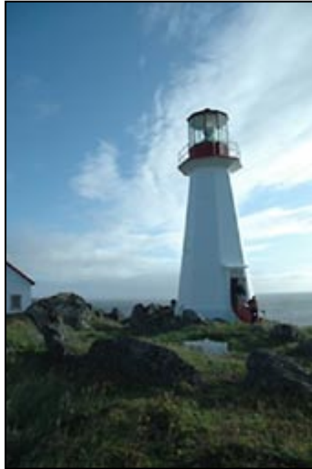
Quirpon Island Lighthouse
